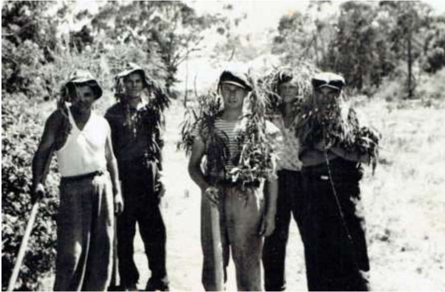
Left: Clearing for a Ballarat Water Commission pipeline: 1951: Kaz Ciężki is third from left.
